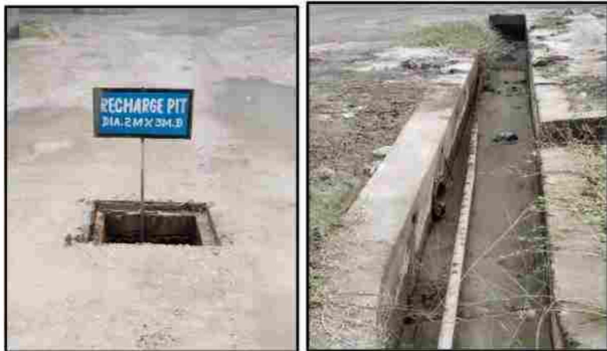
(6) Rain water recharge pit near packing plant covered with chamber and its connecting drainage
