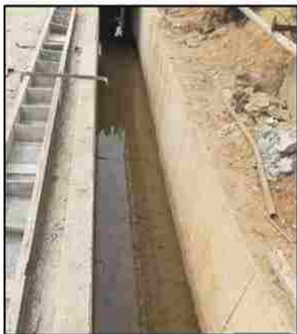
Garland drains and collection pit constructed
