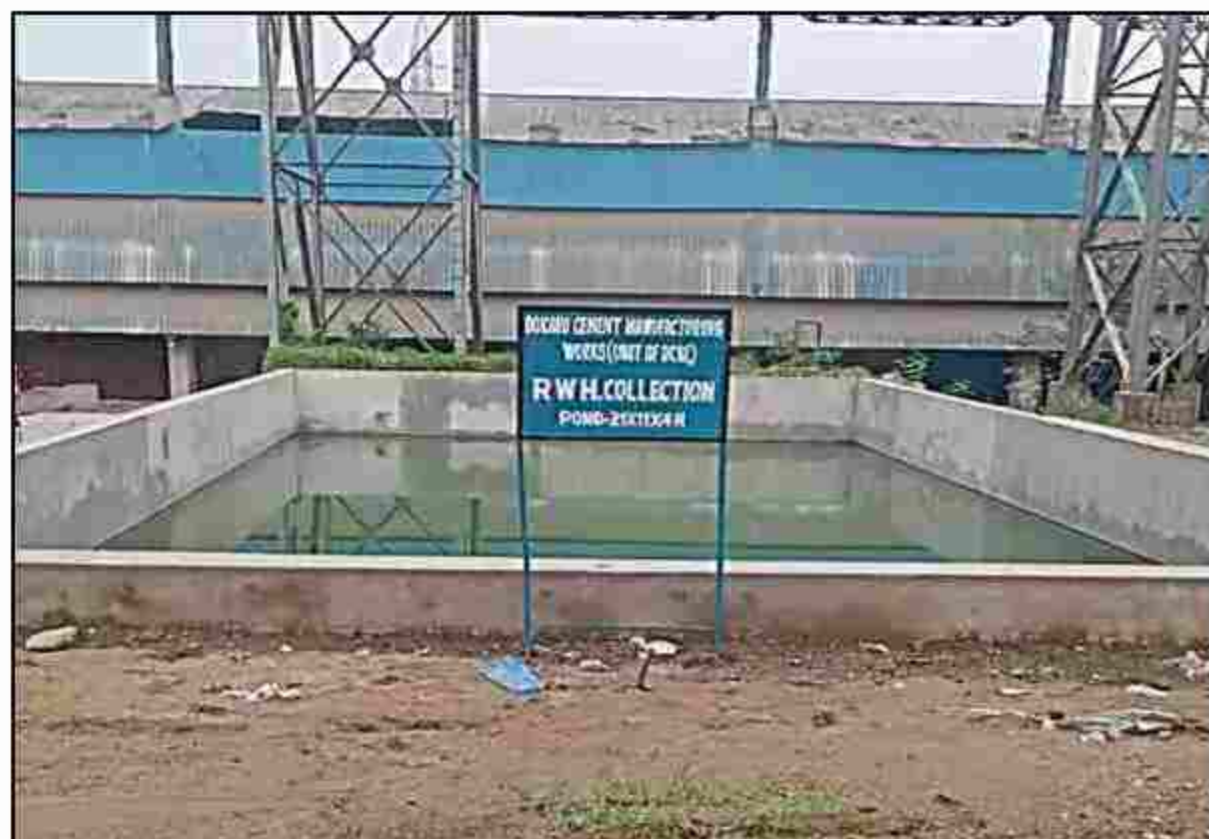
Rain Water collection Pond constructed Capacity: 925 KL
