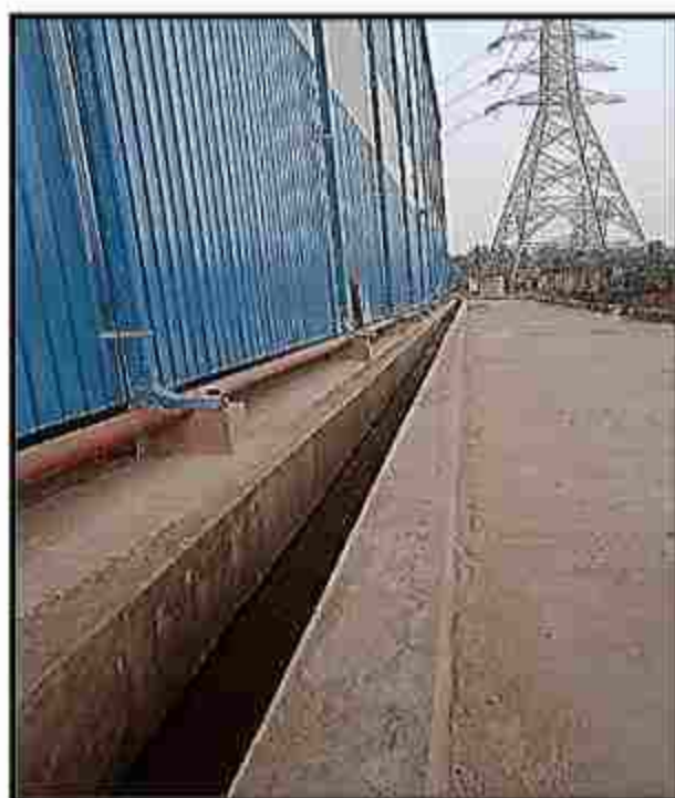
(5) Rain water harvesting pit with Connecting drainage near stacker reclaimer
