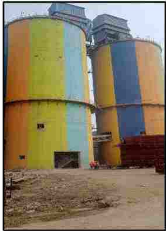
Cement storage Silo
