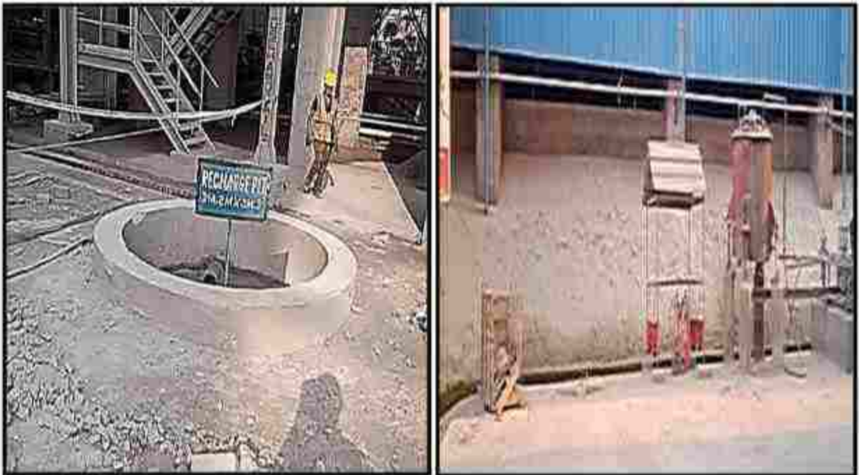
(4) Rain water recharge pit with connecting drain near mill area
