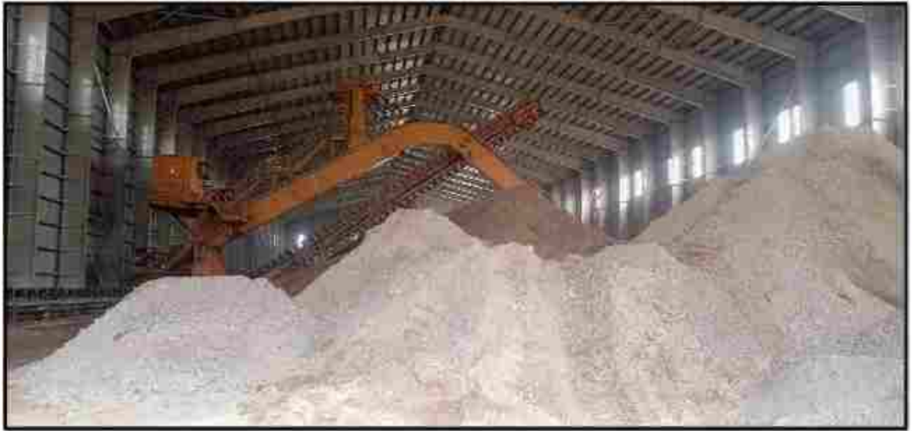
Gypsum stored in covered yard
