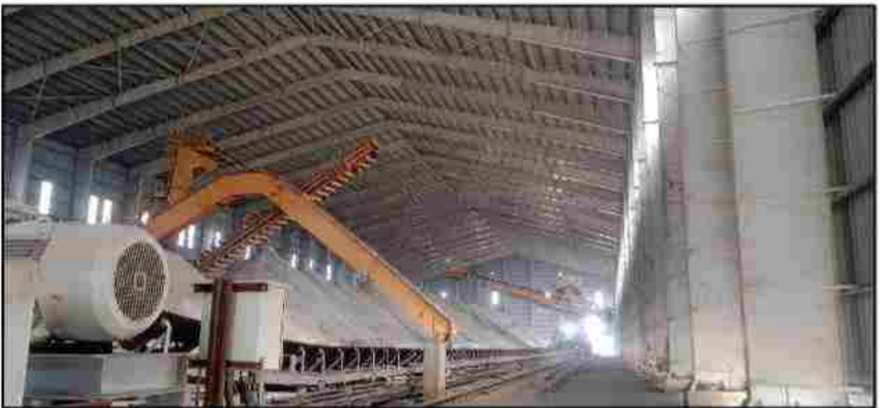
Slag storage in covered yard
