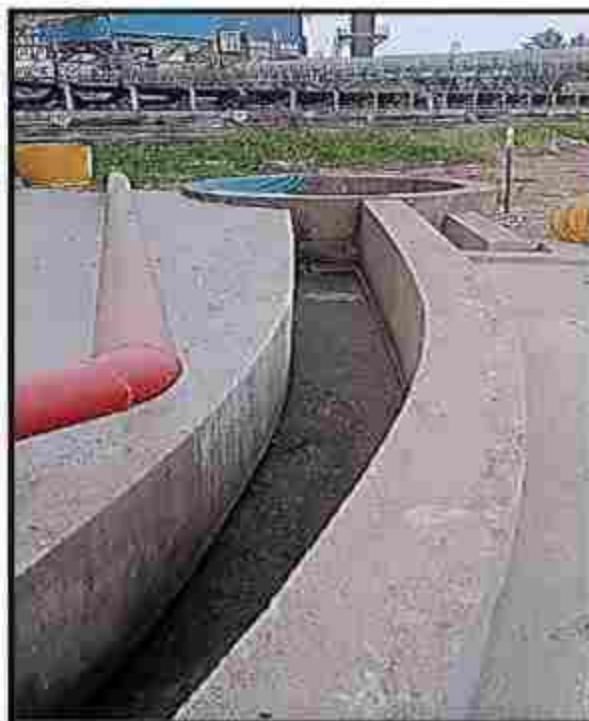
(5) Rain water harvesting pit with Connecting drainage near stacker reclaimer
