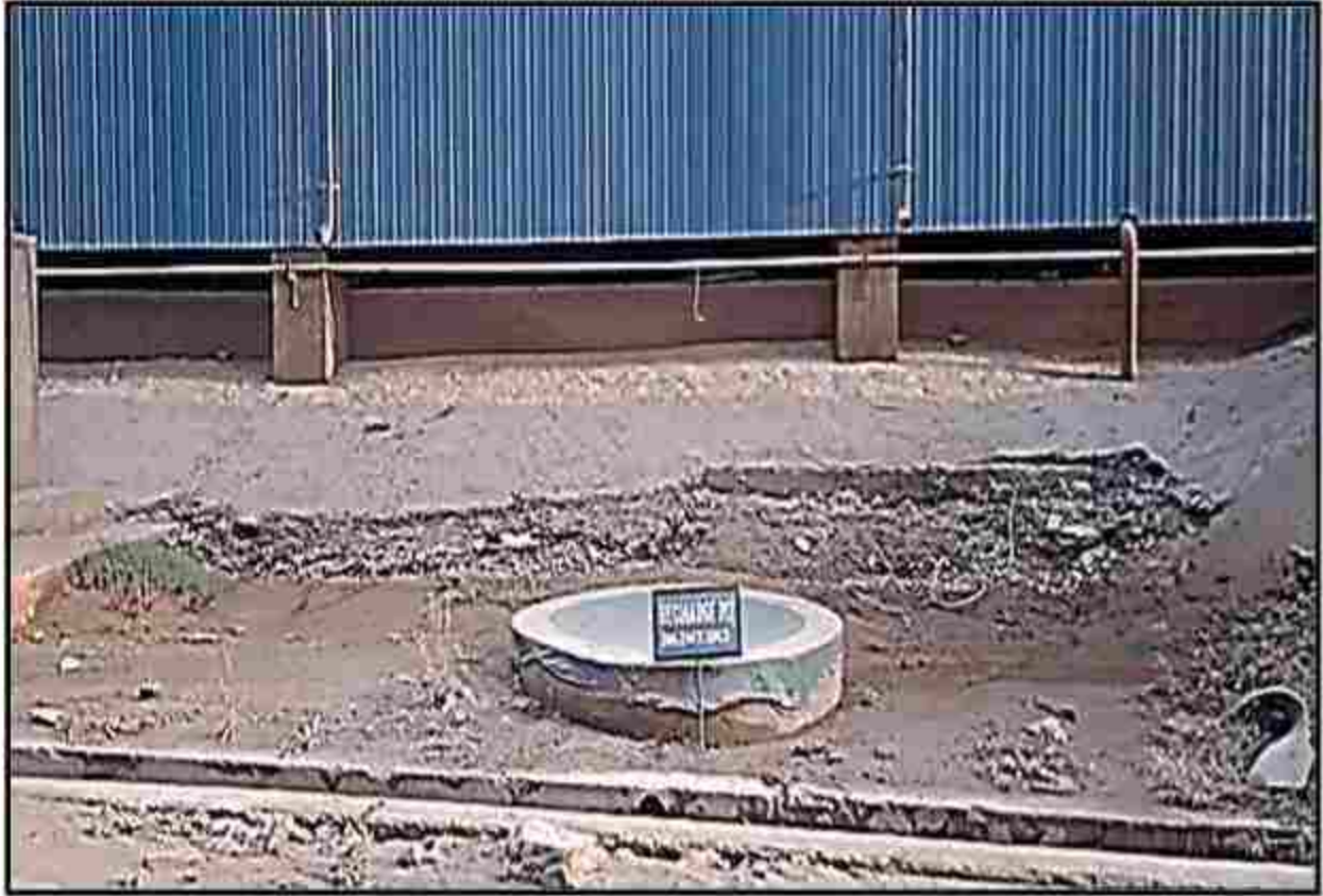
(3) Rain Water Recharge Pit with connecting drain near stacker reclaimer
