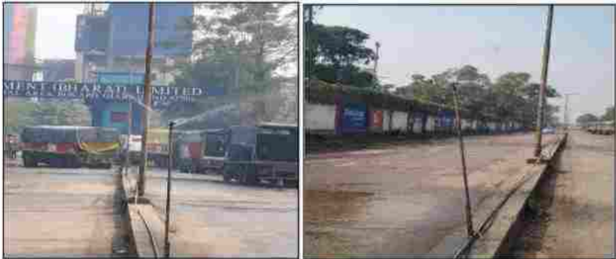
Fixed type water sprinkler installed plant main gate entrance road
