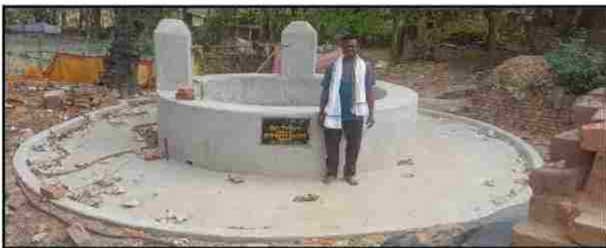
Well renovation for the conservation of water
