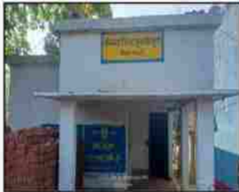
Renovation of Aganwadi
