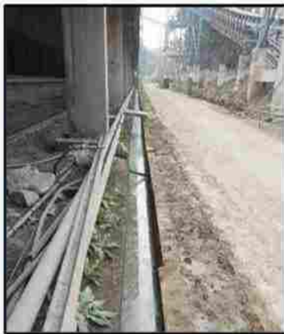
Garland drains and collection pit constructed
